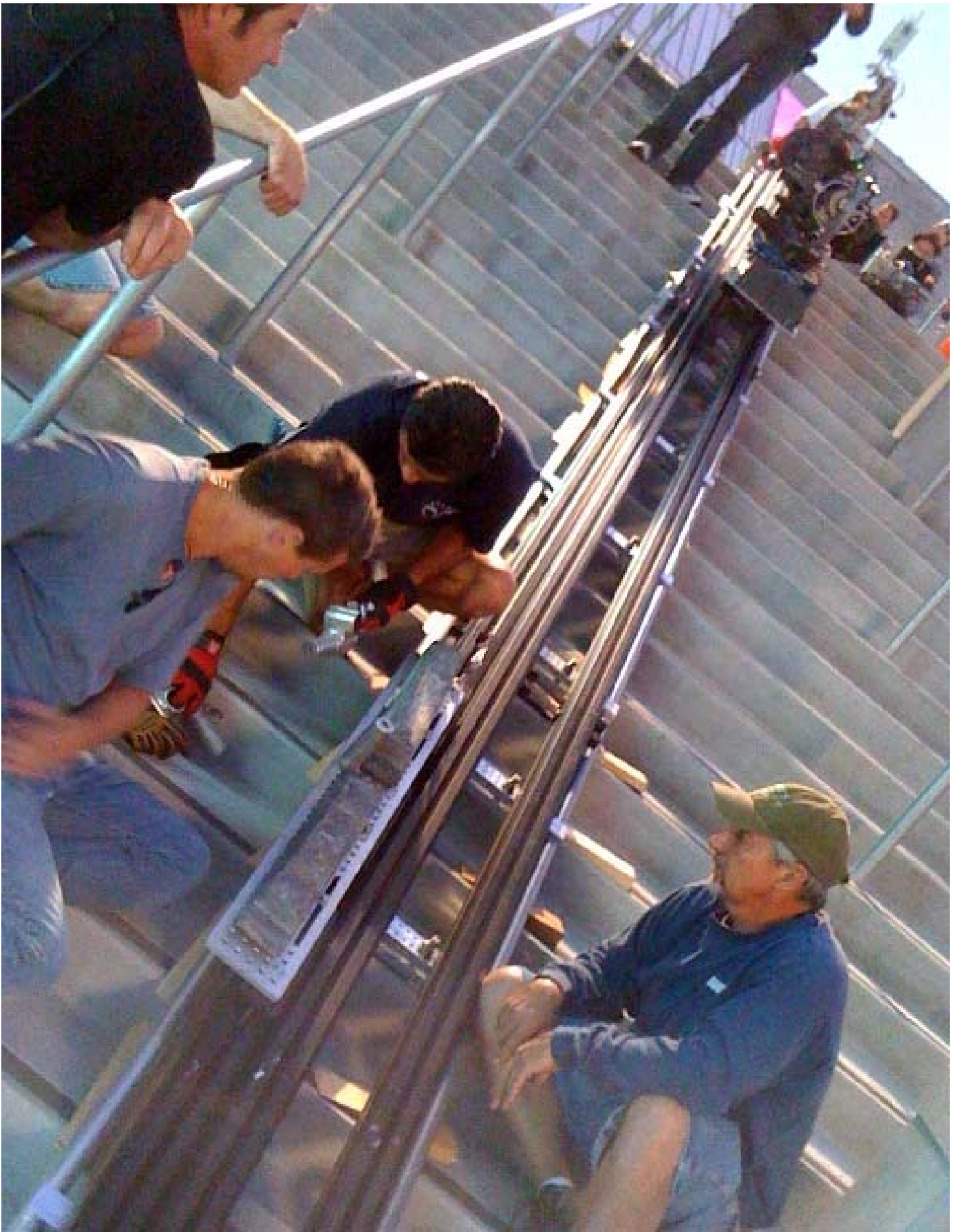
Fastrack grappled to low-profile ladder truss with a counterweight for hand operation.
